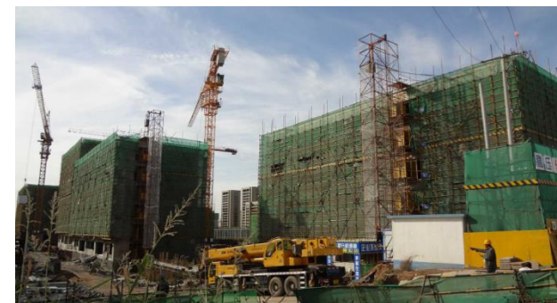
Apartment Site in Shenyang
