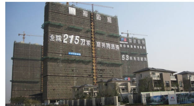
Site of condominium building in
