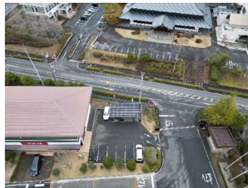
Solar car port at Tsuyama Showroom
