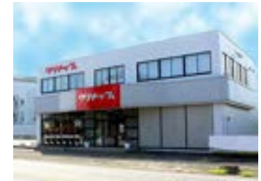
“Komaki Showroom” Reopened after renovation. September 26 (Saturday)
