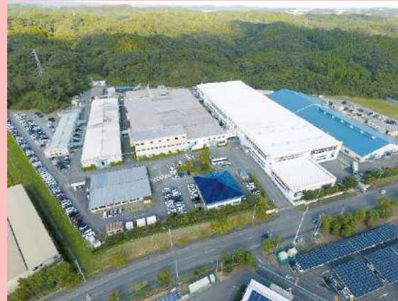
Kashima System Factory (Operations starting in August 2024)
